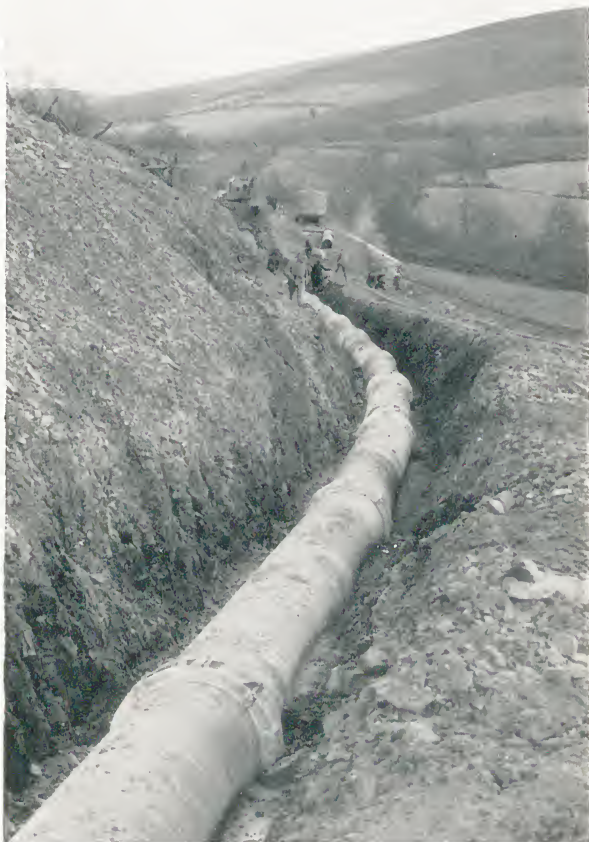
'S & L' steel water main with Viking Johnson Couplings, showing how the flexibility of the Coupling allows a pipeline to be laid in a curve without the use of bends.
